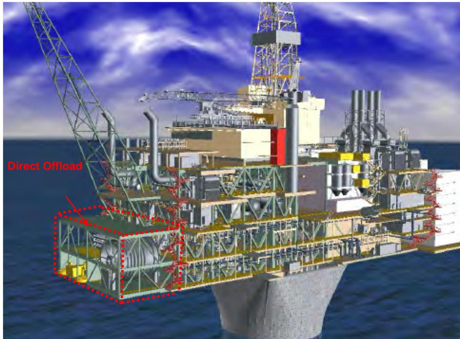
Figure 2-9 Platform Location of Direct Offloading Equipment
